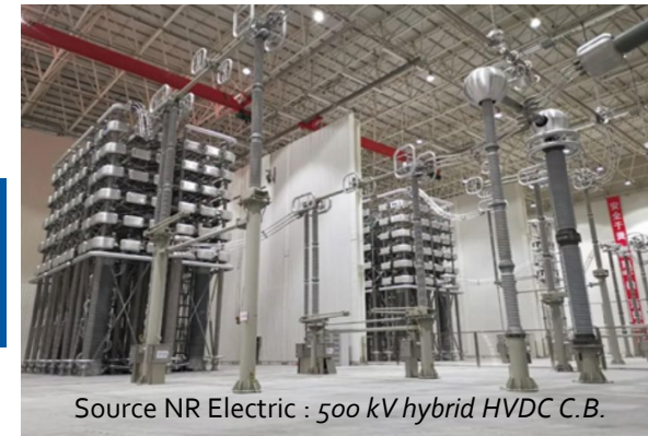
HVDC Circuit Breaker Active Current Injection Technology
